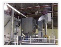
DustHog SFC 32-4 with Safety Filter used for blending powdered cheese, baking mixes and tortillas.
