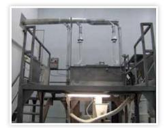
Stainless ducting is used with this dump station. Ducting is attached to DustHog SFC 32-4 above.
